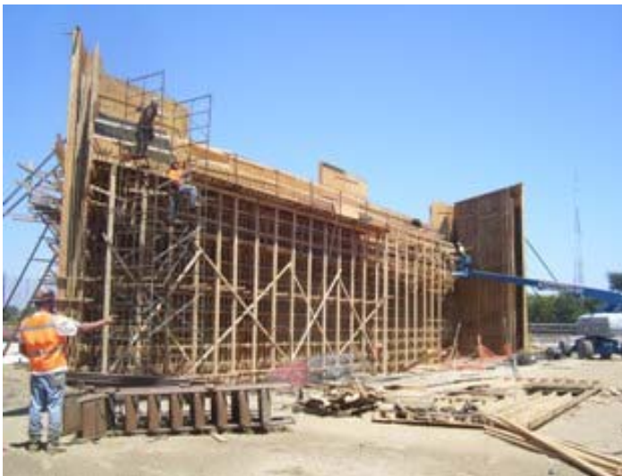
Photo above and right: 5 th Street bridge foundation form and rebar work.
