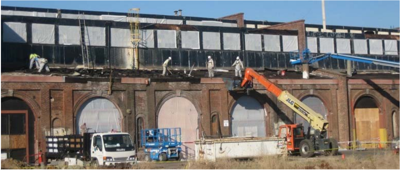
Photo above: Allied Environmental working on Car Shop No. 3.
