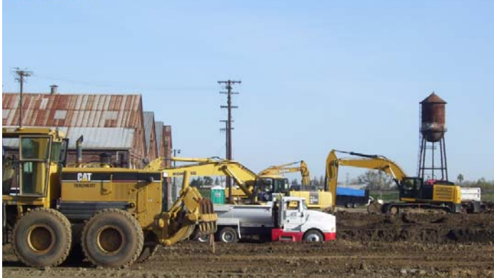
Getting the Main Line Tracks Area Ready March 26, 2010
