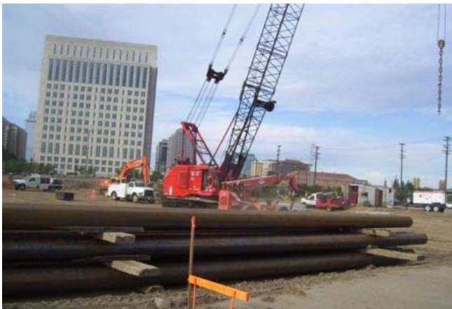
Photo above: Pile driving preparations in progress.
