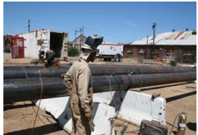
Photo above: Pile welders at work.
